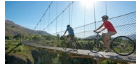
Edgar Bridge on the Arrow River Trail
